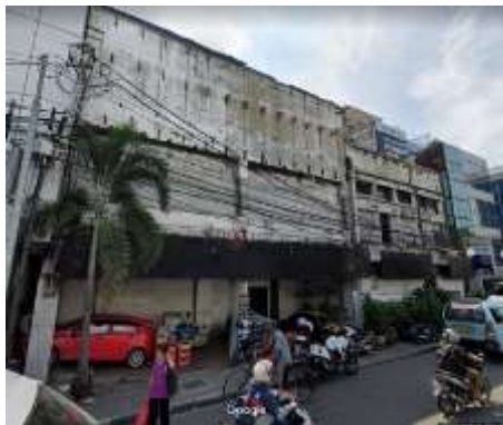
Gambar 3.5 View Existing Entrance 3 (Sumber: Dokumentasi PT. Hutama Karya)
