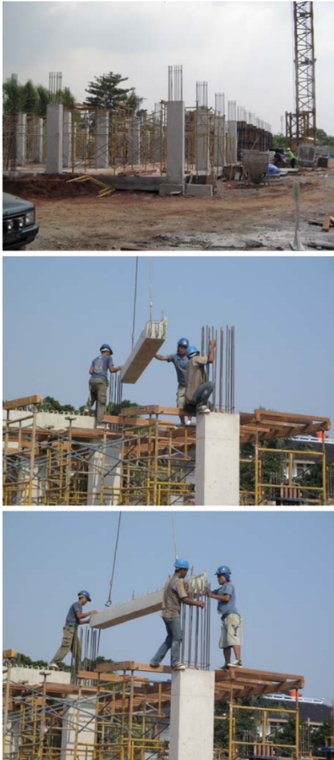
Fig. 1. Erection process the precast system.
