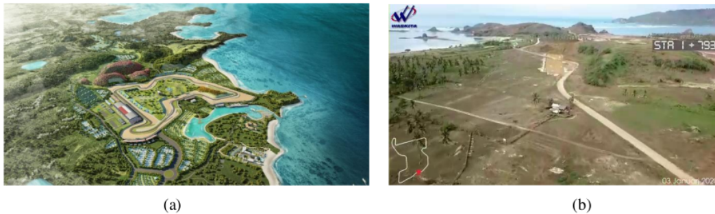
Fig. 1– (a) Map of Mandalika MotoGP circuit, Lombok, (b) Construction progress of Mandalika Moto GP circuit, Lombok
