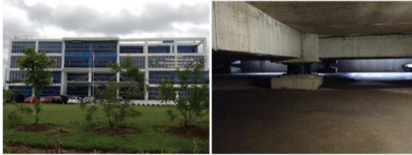
Fig. 18 – Seismic Bearing Installation
