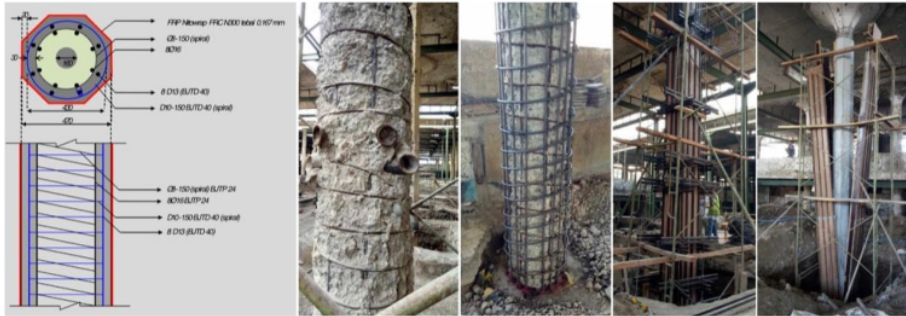
Fig. 11 – Concrete Retrofitting Design & Process
