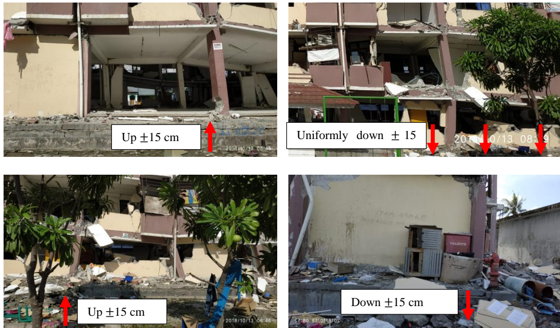
Fig. 2 – Soil deformation pattern due to vertical earthquake (pictures continuous along the length of building)
