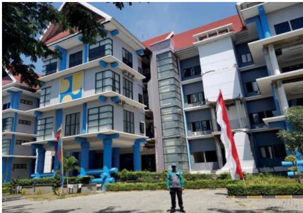
Fig. 2 – Damage in the Front of the Building
