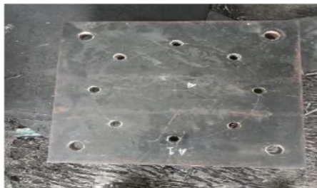
Drill an no penetrate hole to attach the countersunk bolt that secures the flange plate to the LRB body
