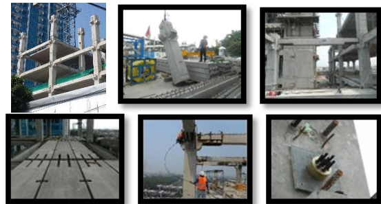
Figure 15. Twelve storey Tamansari Office Hive (2015)
