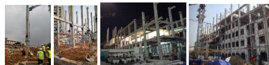
Figure 16. Six-storey Apartment in Jakarta (2015)
