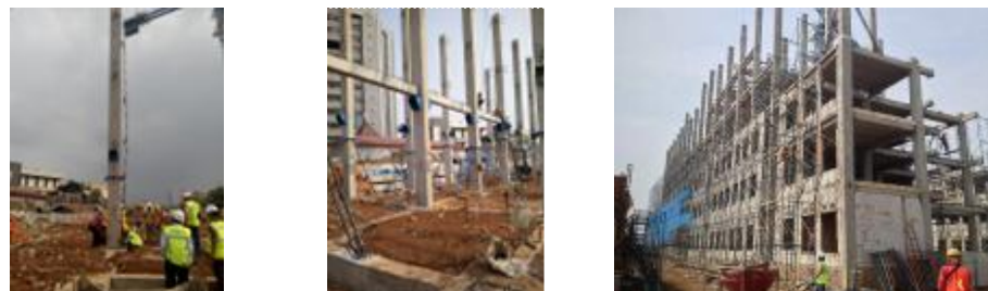
Fig.20 – Application in multistorey low cost housing in Jakarta
