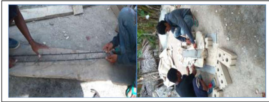
Figure 5 Construct concrete reinforcement for latei-beam
