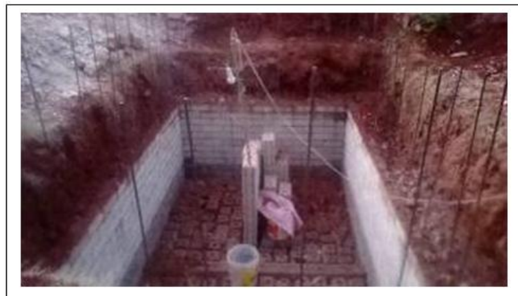
Figure 9 Installation of pond wall
