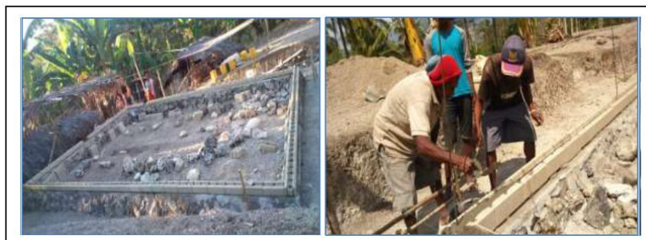
Figure 2 Foundation and installing iron on the sloof beam.
