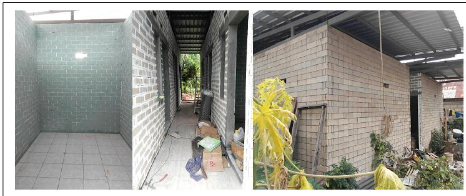
Figure 11 Student dormitory building using lock-brick system
