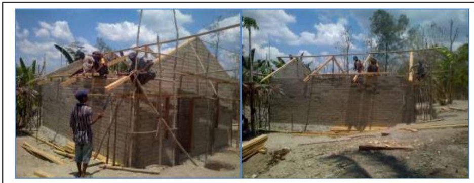
Figure 6 Implementation of roof installation work
