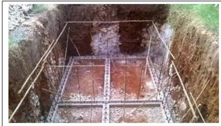
Figure 8 Installation of sloof beam reinforcement floors of pond..
