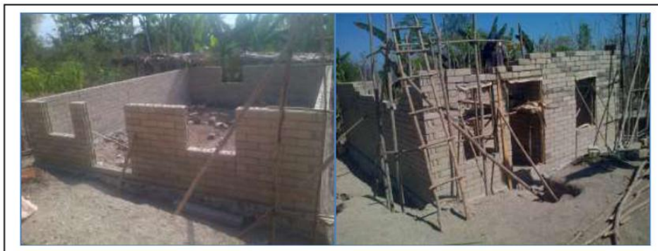
Figure 4 Installation of lock-brick wall, door and window holes
