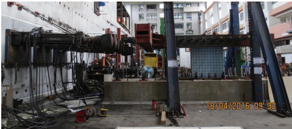
Figure 2 SC wall test setup
