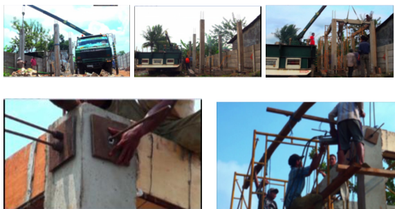
Fig. 7 First building using PRESSS
