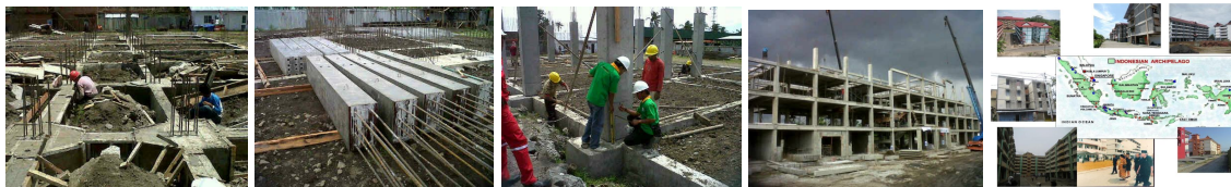
Figure 2.2. Construction of low cost housing with precast concrete system
