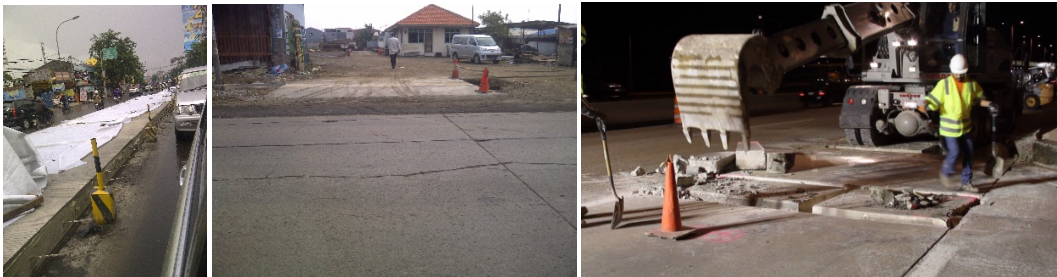
Figure 1 Conventional rigid pavement (JPCP)
