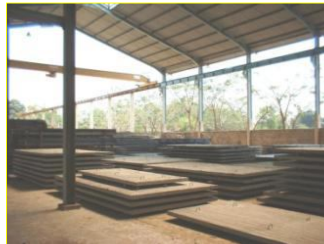
Half slab beton bertulang
