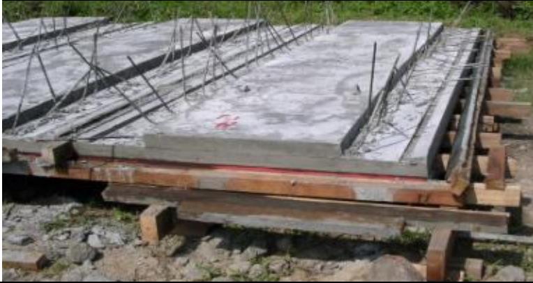
Proses demolding
