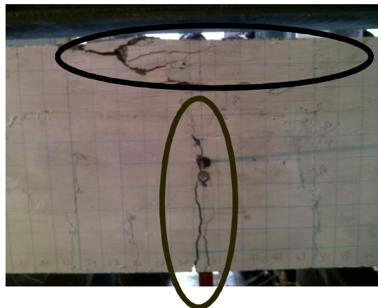
1% - Tension Gap at Dissipater and compression failure
