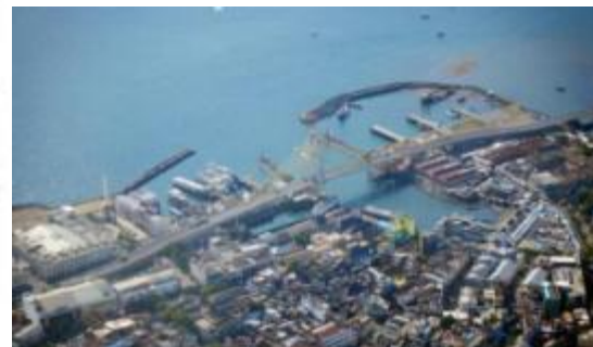
Soekarno Bridge, Manado (2015)
