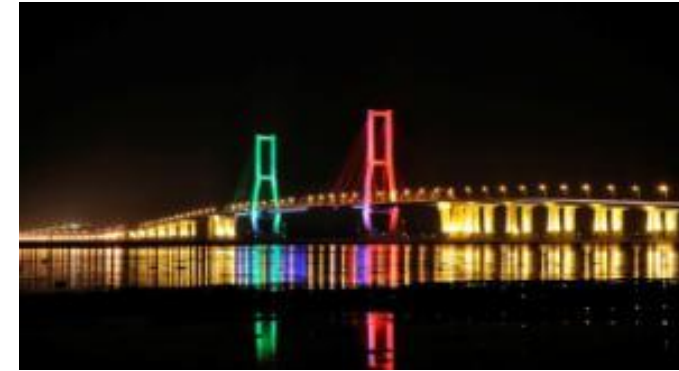
Suramadu Bridge, Surabaya (2009)
