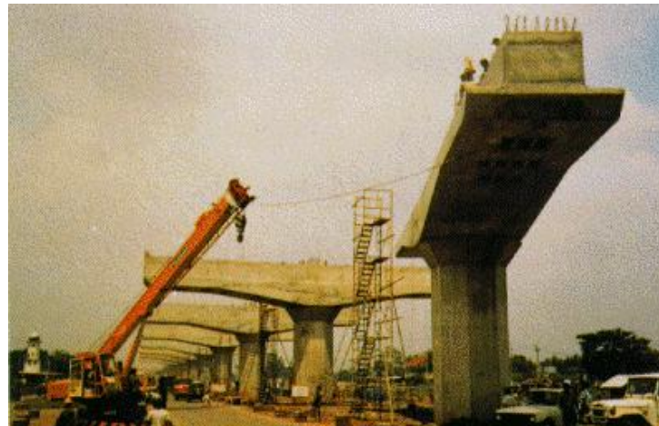
Tiang Pancang, Girder, Sosrobahu Jalan Lavang Cawang-Priuk 1985
