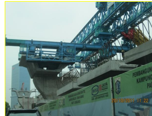
Alat erection Launcher
