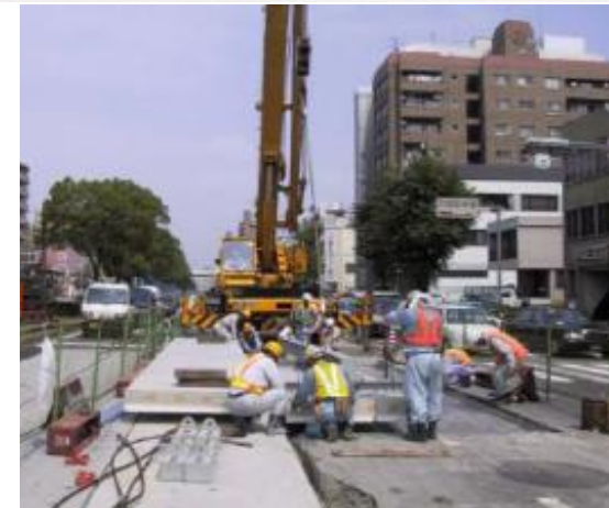
Precast Rigid Pavement
