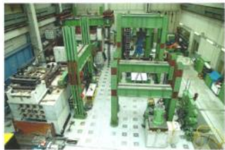
14 x 24 m 2 strong floor for variable testing of structural members
