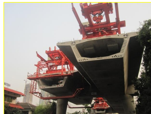
Alat erection Lifter
