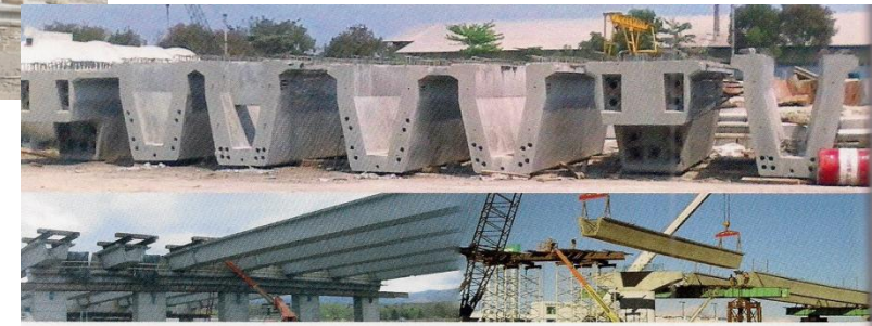
Industri Beton Pracetak dan Prategang Start in 1974 with Precast Government Company Bridge
