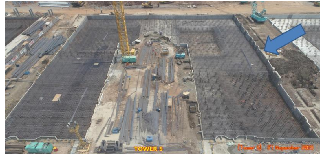
Precast Retaining Wall For Raft Foundation
