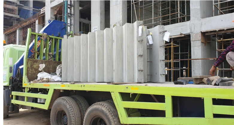
Precast Stair Case
