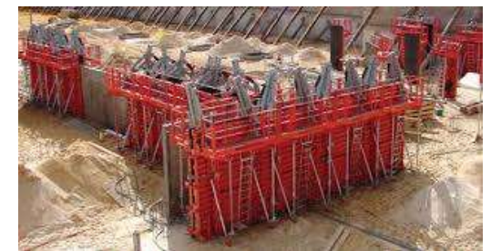
Sistem Formwork Bearing Wall
