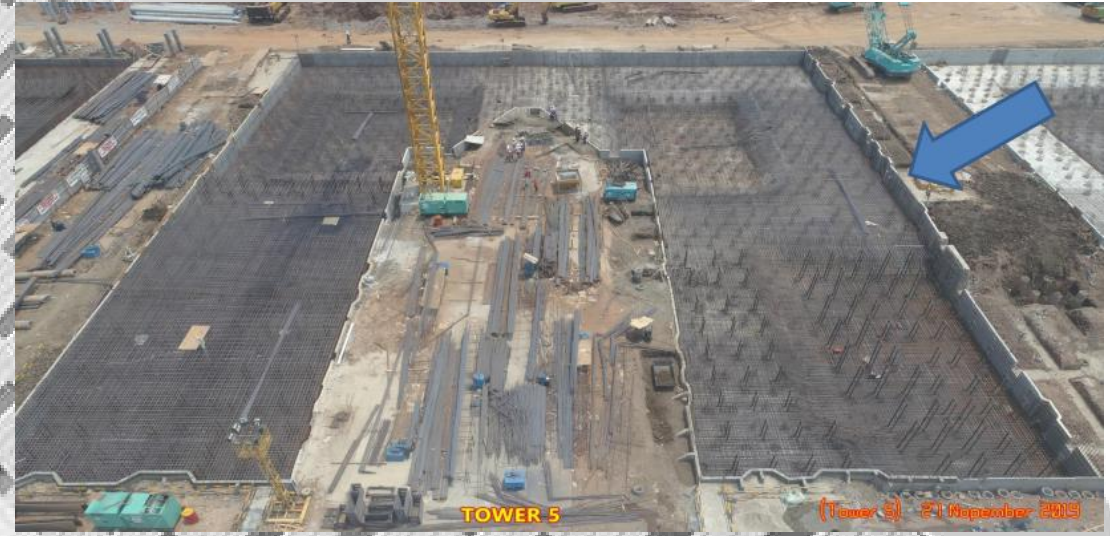
Precast Retaining Wall For Raft Foundation
