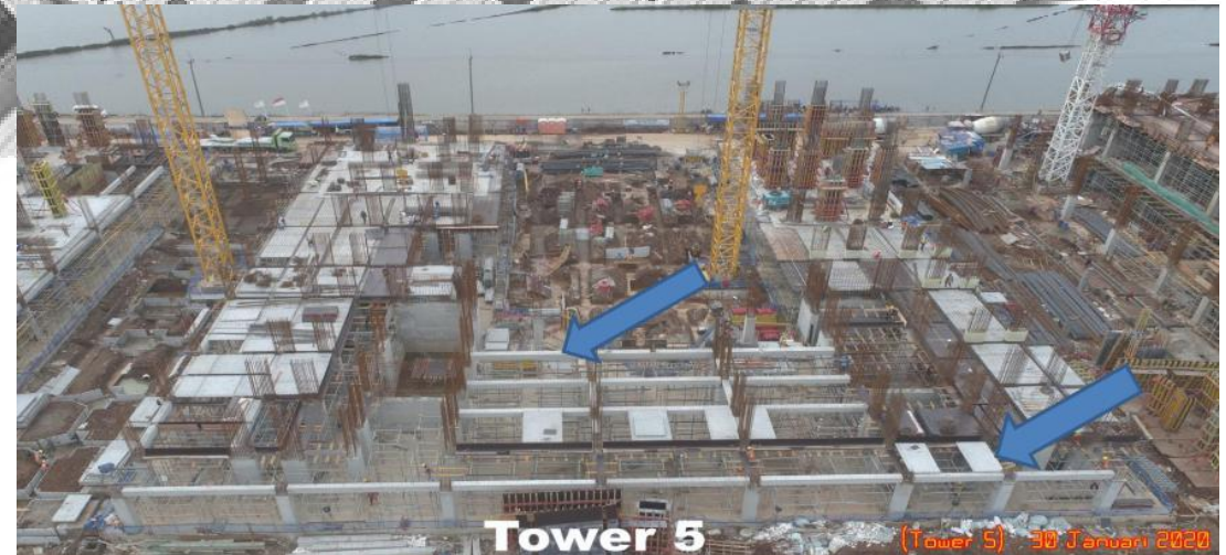
Beam, Half Slab Precast System
