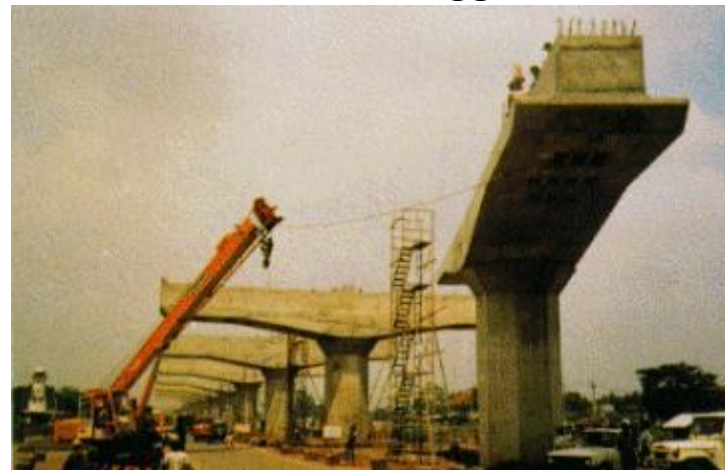
Tiang Pancang, Girder, Sosrobahu Jalan Lavang Cawang-Priuk 1985
