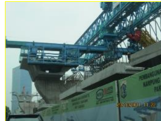
Alat erection Launcher
