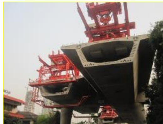
Alat erection Lifter
