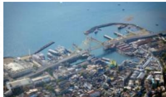
Soekarno Bridge, Manado (2015)
