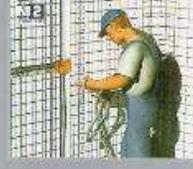
Rigid or semi-rigid pipes for public services (electricity, water, gas, etc.) are easily placed behind the wire mesh.
