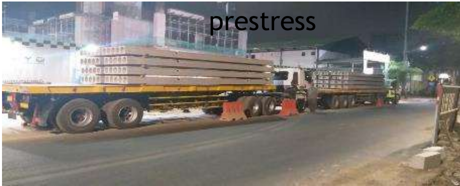
Offsite construction komponen hollow core slab
