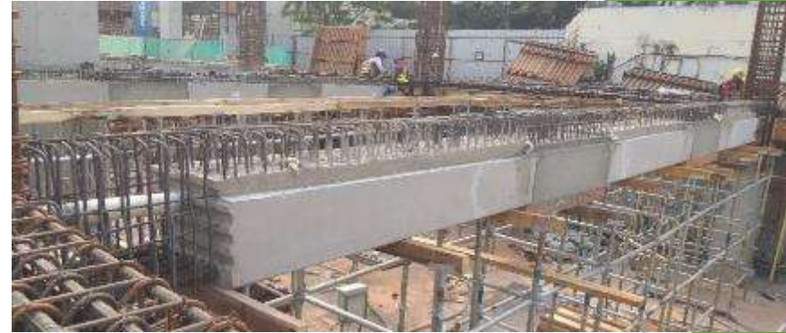
Offsite construction komponen balok precast prestress
