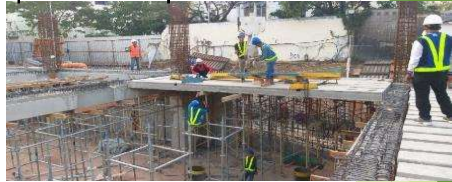
Offsite construction komponen hollow core slab
