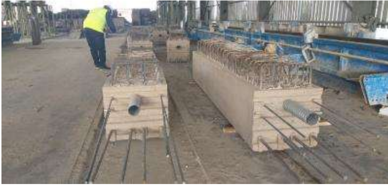
Offsite construction komponen balok precast prestress
