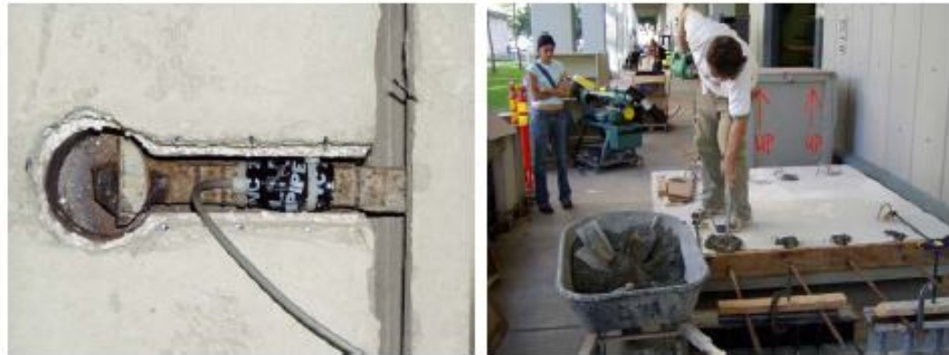
Figure 1-2: Kwik Joint coupler male component
