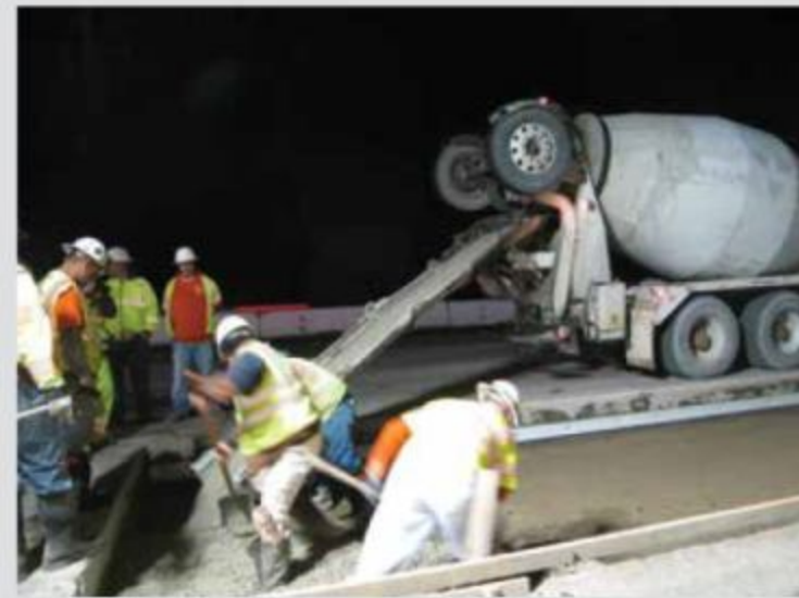
Figure 6. Placing and grading lean concrete base.
