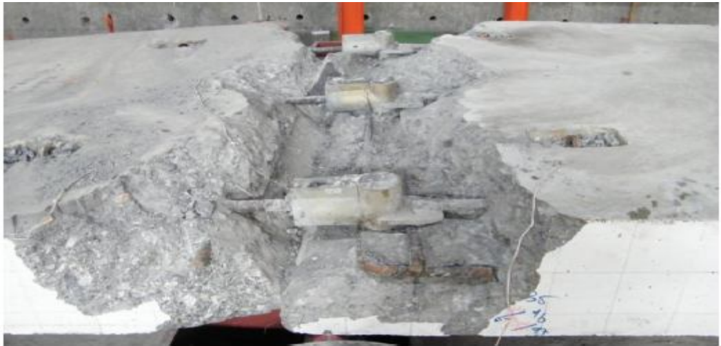
Figure 4.22 Condition of Kwik Joint at Flexural Test Specimen
