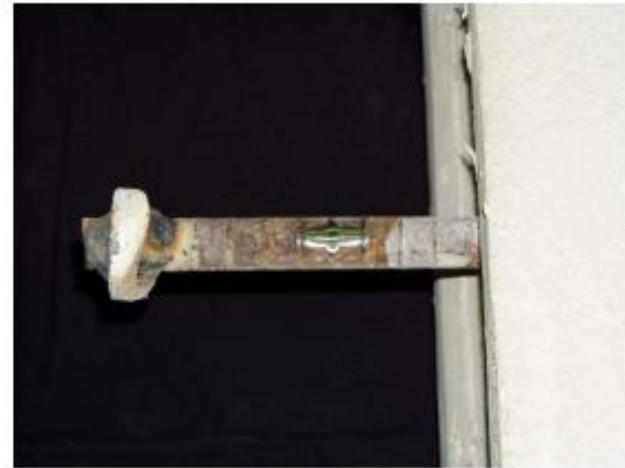
Figure 1-2: Kwik Joint coupler male component
