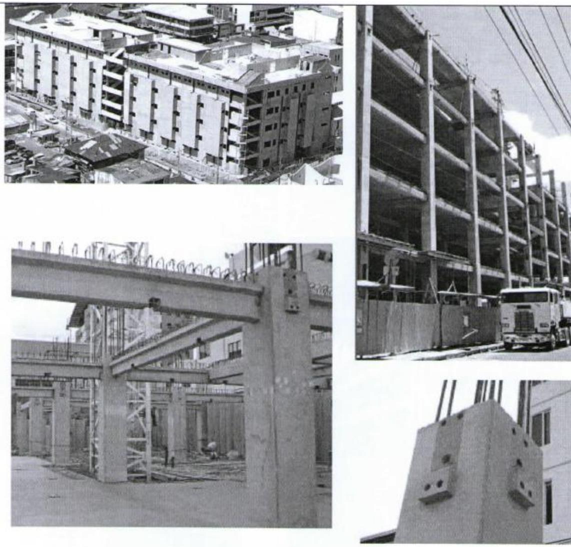
**Figure 10.5 - Clínica Bíblica Hospital, downtown San José, Costa Rica. Two underground stories and Five stories above the ground. Designed to remain operative after an extreme earthquake event (photo courtesy of Productos de Concreto, Holcim Costarica)**
