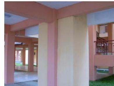
(a) Earthquake at March 6, 2007, there is architecture damage in 1<sup>st</sup> floor, no structural cracks
