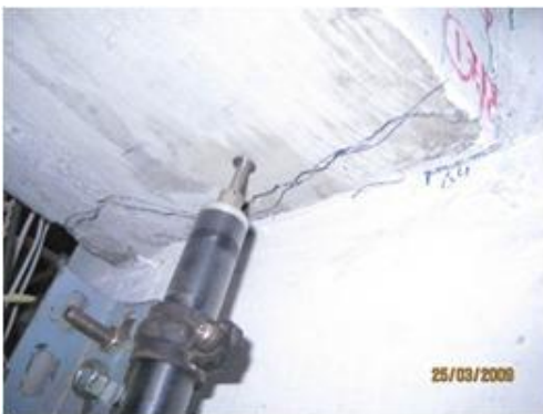
(b) Earthquake at September 30, 2009, heavier architecture damage and structural cracks on 1st floor
