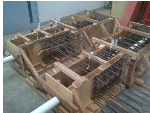
Pemasangan ducting unbonded
