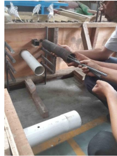
Pemasangan ducting unbonded
