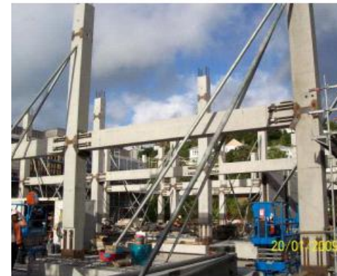
EXTERNAL DISSIPATERS: mild steel rods with epoxied encased steel tubes
