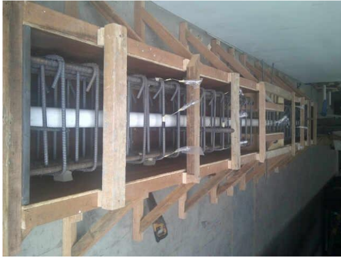
Pemasangan ducting unbonded
