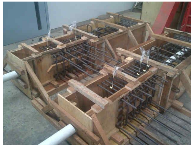
Pemasangan ducting unbonded
