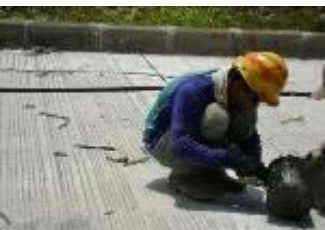
Underslab grouting, siap berfungsi 8 - 48 jam
