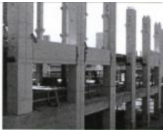
Figure 25 Five-Storey PRESSS Building tested at University of California, San Diego [13]
