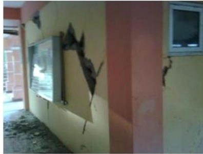
(b) Earthquake at September 30, 2009, heavier architecture damage and structural cracks on 1st floor
