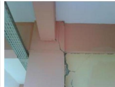
(b) Earthquake at September 30, 2009, heavier architecture damage and structural cracks on 1st floor
