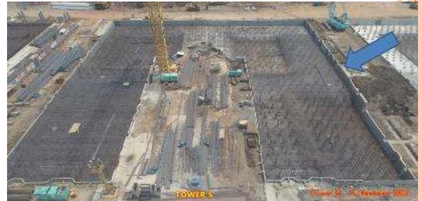
Precast Retaining Wall For Raft Foundation
