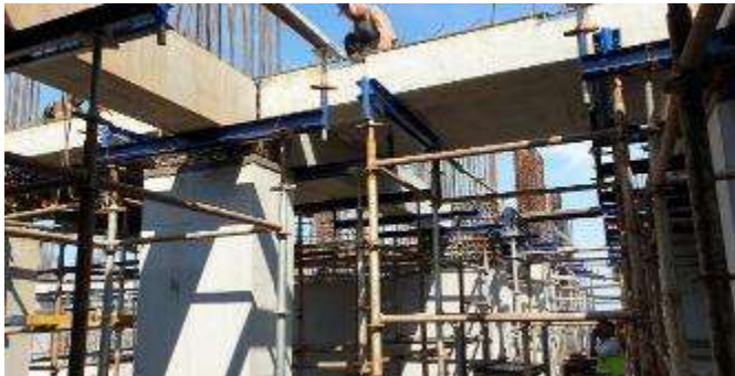
Beam Installation
