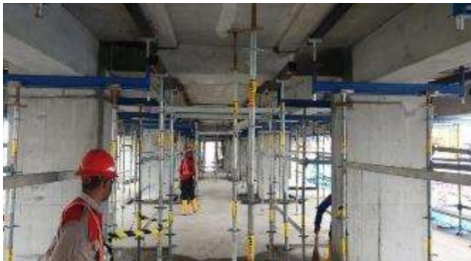
Beam Installation
