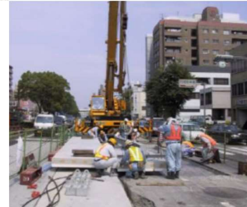
Precast Rigid Pavement
