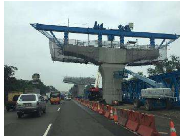
PRECAST POST TENSION SEGMENTAL PIER HEAD
