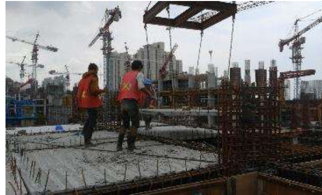
Erection slab precast
