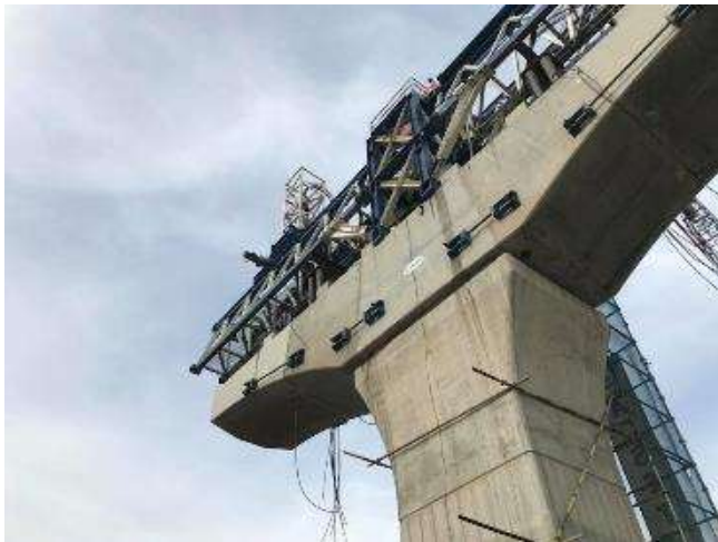
PRECAST POST TENSION SEGMENTAL PIER HEAD
