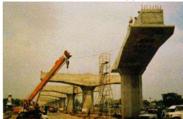
Tiang Pancang Girder, Sosrobahu Jalan Lavang Cawang-Priuk 1985
