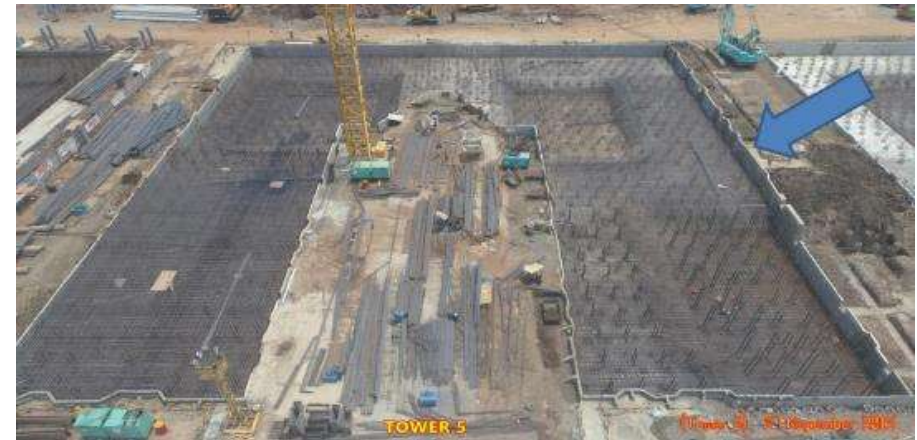
Precast Retaining Wall For Raft Foundation
