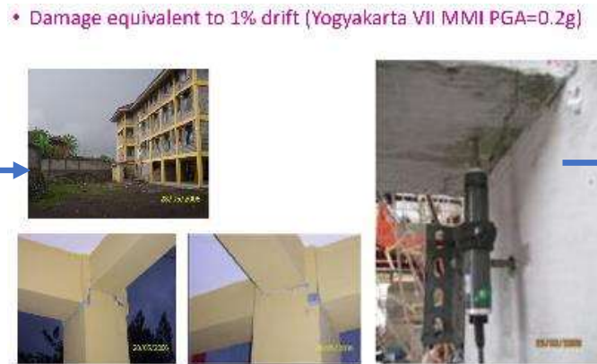
This building have soft story effect (old design before 2008)
