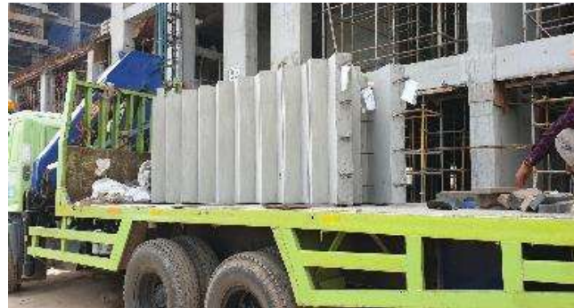
Precast Stair Case
