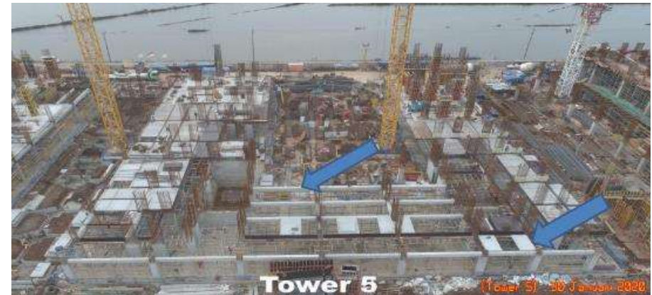
Beam, Half Slab Precast System
