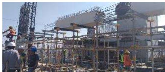
Balok segmental long span dan hollow core slab off site.
