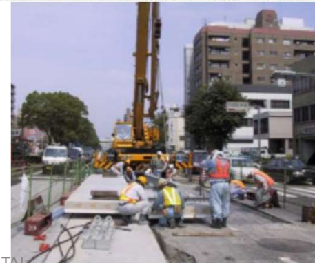
Precast Rigid Pavement
