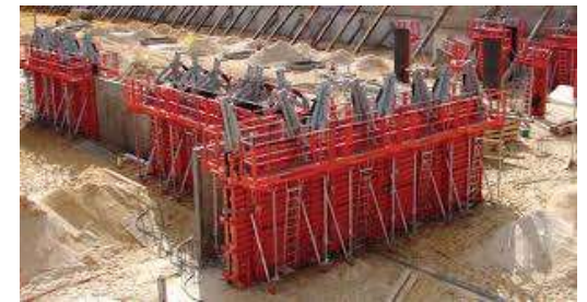
Sistem Formwork Bearing Wall
