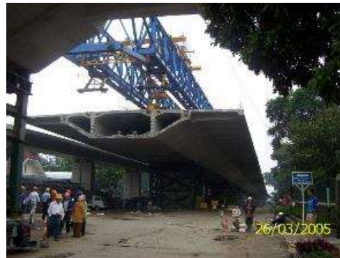
5. Erection - Stressing
