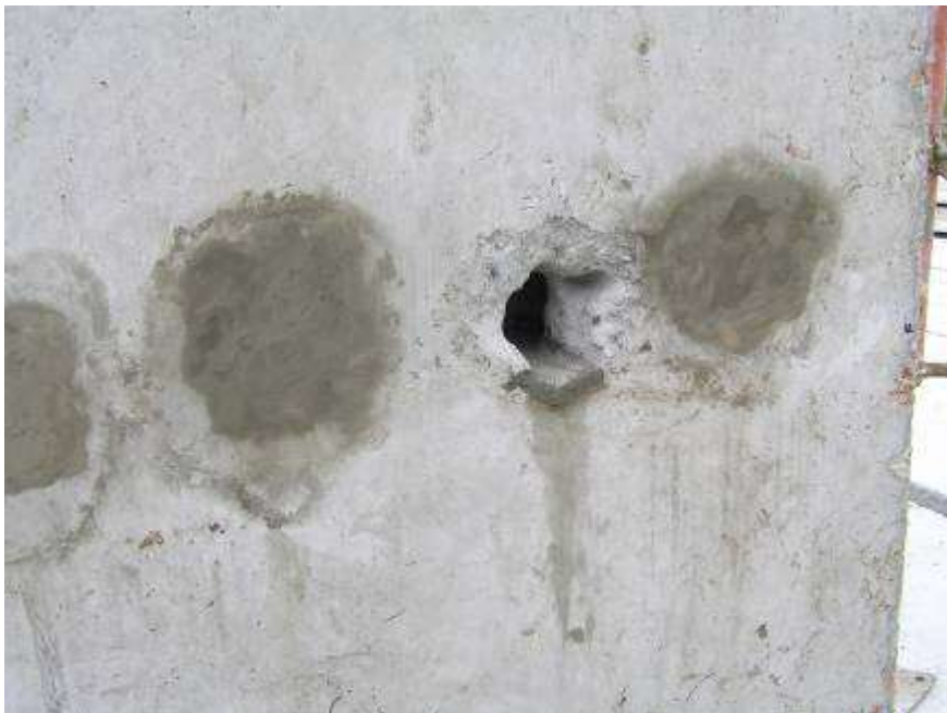
Pengecoran grouting angkur
