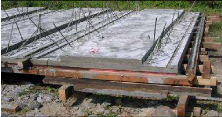
Proses demolding
