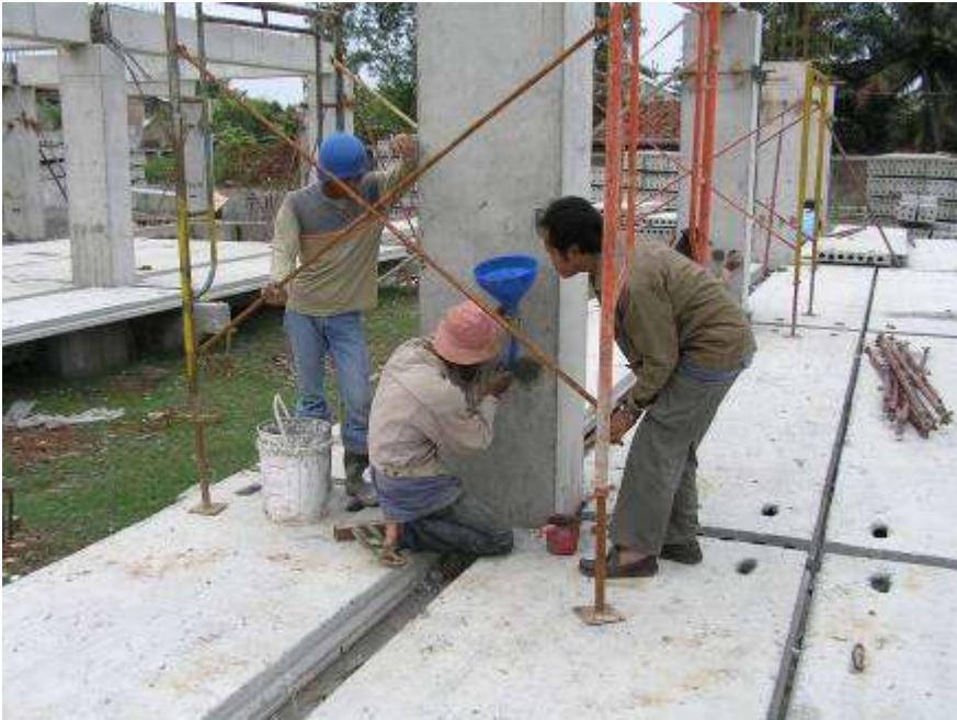
Pengecoran grouting angkur
