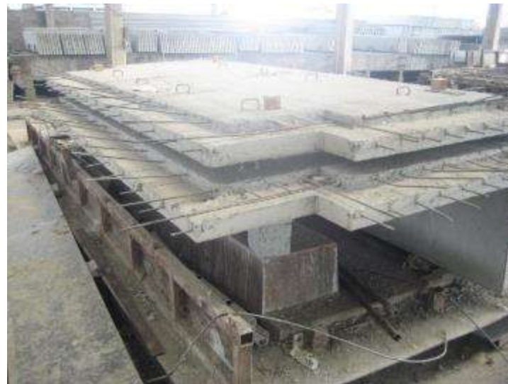
Full slab beton prategang
