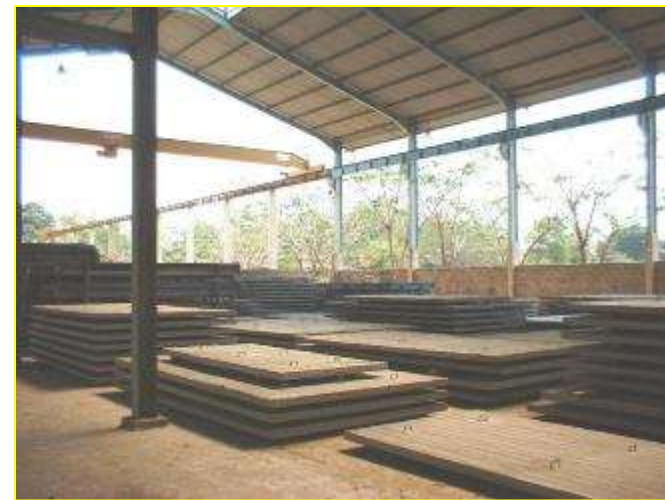
Half slab beton bertulang
