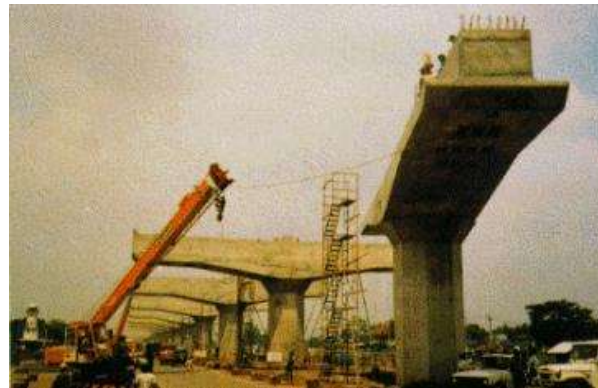
Tiang Pancang Girder, Sosrobahu Jalan Lavang Cawang-Priuk 1985
