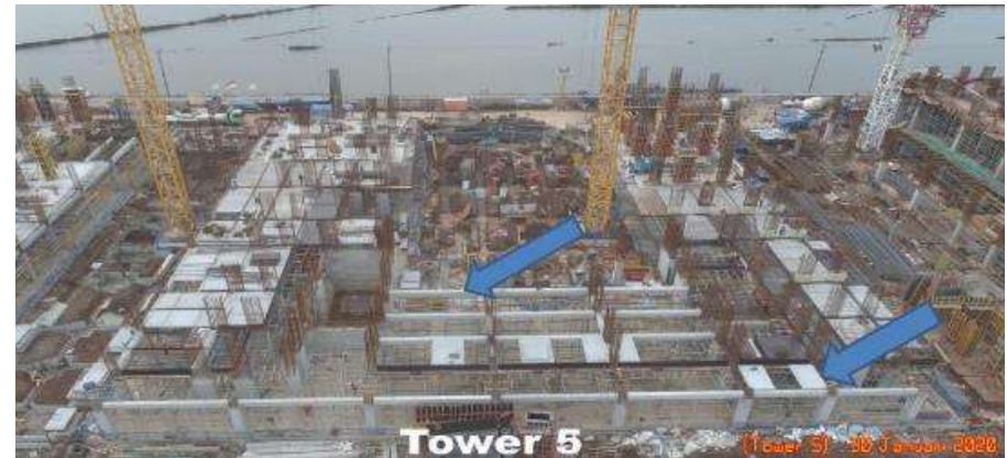
Beam, Half Slab Precast System
