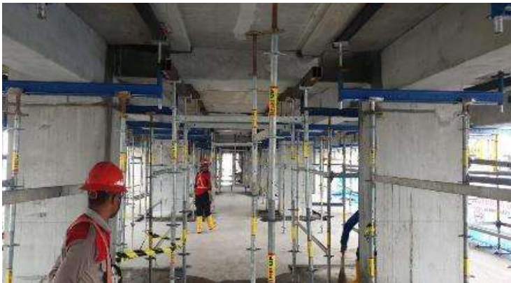
Beam Installation
