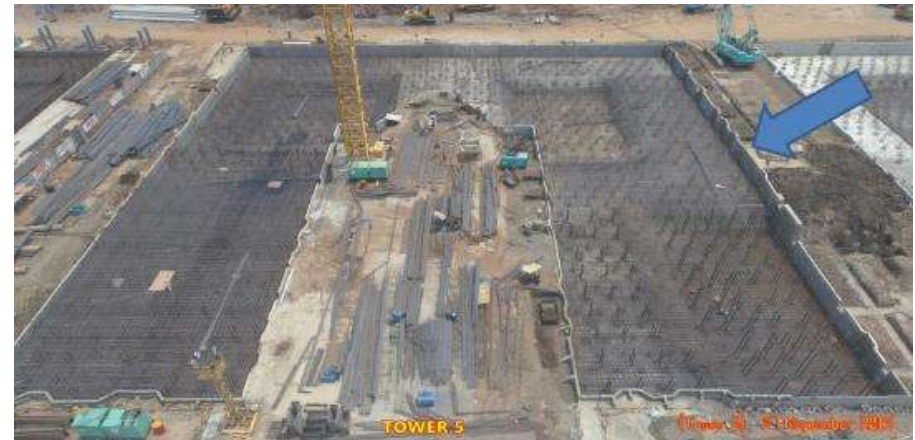
Precast Retaining Wall For Raft Foundation
