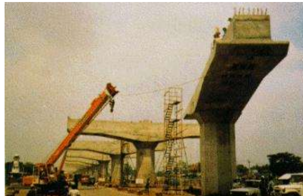
Tiang Pancang, Girder, Sosrobahu Jalan Lavang Cawang-Priuk 1985
