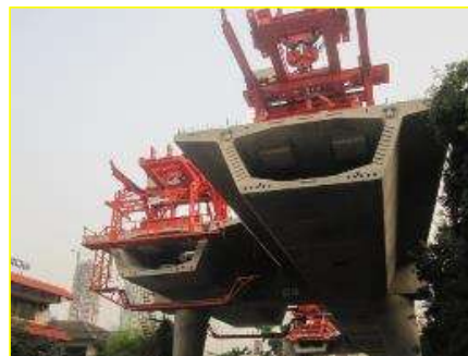
Alat erection Lifter
