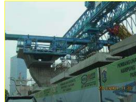
Alat erection Launcher
