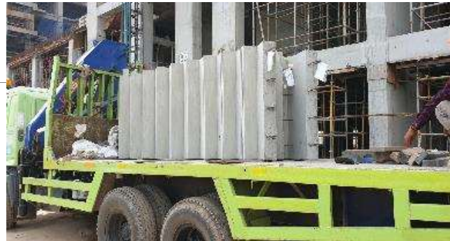
Precast Stair Case
