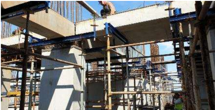
Beam Installation
