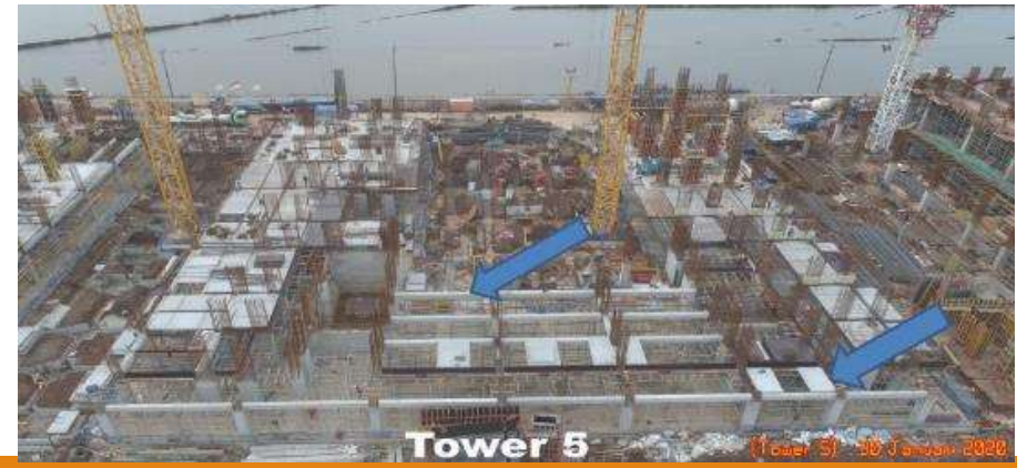
Beam, Half Slab Precast System
