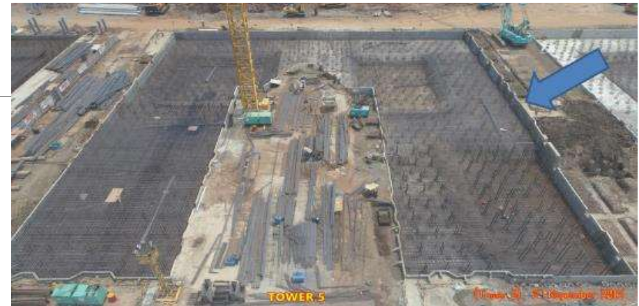
Precast Retaining Wall For Raft Foundation
