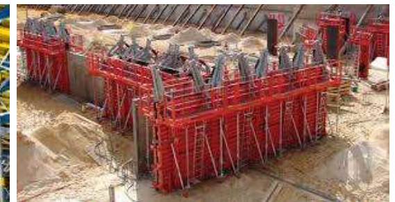
Sistem Formwork Bearing Wall
