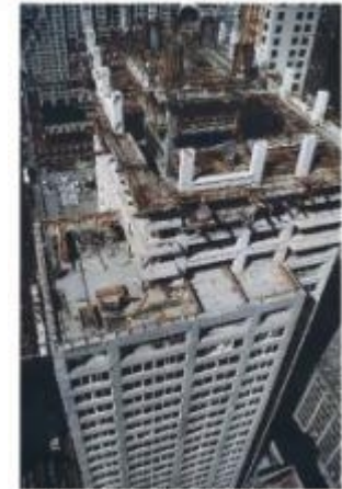
Fig. 21. Installation of precast concrete. Drawing courtesy: Sean Florko, Architect and Planning.
