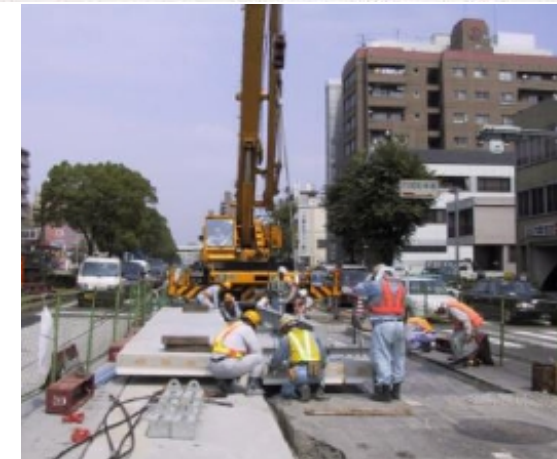
Precast Rigid Pavement
