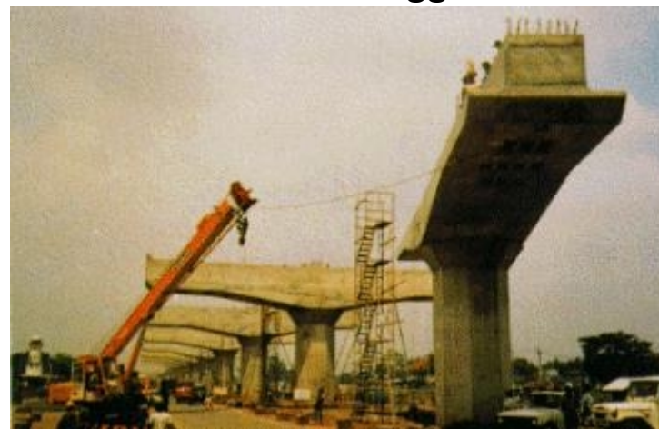
Tiang Pancang, Girder, Sosrobahu Jalan Lavang Cawang-Priuk 1985
