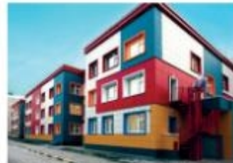
SO-155 is also involved in the social sector with facilities such as kindergartens and schools.
