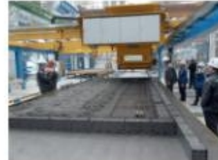
Concreting of the first solid wall elements in Kemerovo
