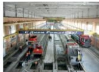
Ehsew Precast Engineering equipped the Domodedovo works of the SO-155 construction group with a production plant for prestressed hollow core slabs.
