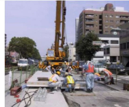
Precast Rigid Pavement
