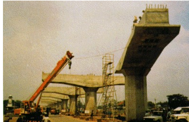
Tiang Pancang, Girder, Sosrobahu Jalan Lavang Cawang-Priuk 1985
