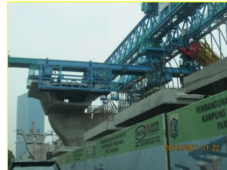
Alat erection Launcher
