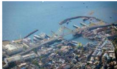
Soekarno Bridge, Manado (2015)
