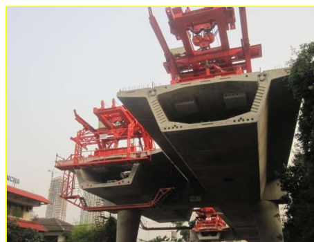
Alat erection Lifter
