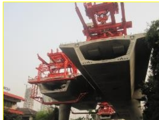
Alat erection Lifter
