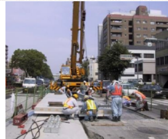
Precast Rigid Pavement
