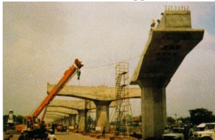
Tiang Pancang, Girder, Sosrobahu Jalan Lavang Cawang-Priuk 1985
