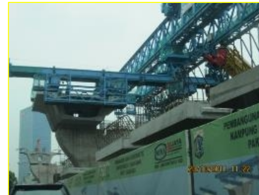
Alat erection Launcher
