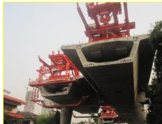
Alat erection Lifter
