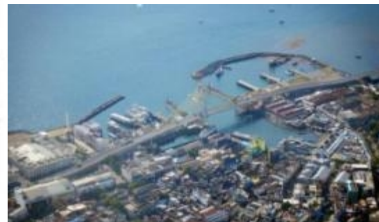
Soekarno Bridge, Manado (2015)
