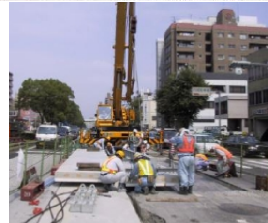
Precast Rigid Pavement
