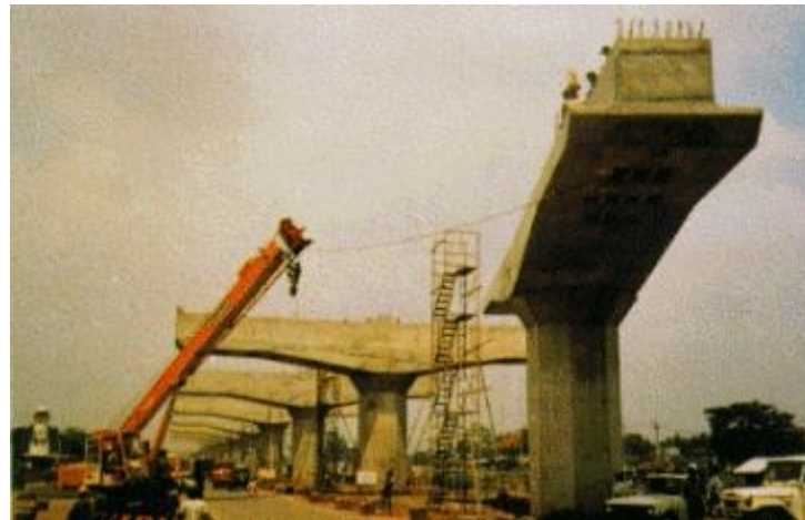
Tiang Pancang, Girder, Sosrobahu Jalan Lavang Cawang-Priuk 1985
