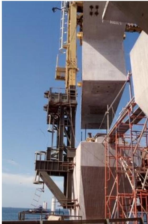
Pier bracket utk aktifasi tumpuan launching gantry saat erection ▼ pier segment.
