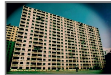
Figure 4. Jalan Pekeliling Flat, Kuala Lumpur
