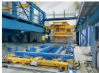
Commissioning of the concrete distributor in KIn – a completely new precast plant is being erected here for the production of sandwich walls as well as solid wall and floor elements.
