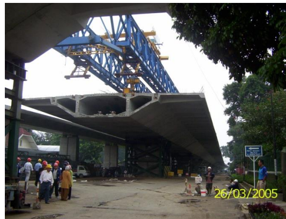
5. Erection - Stressing
