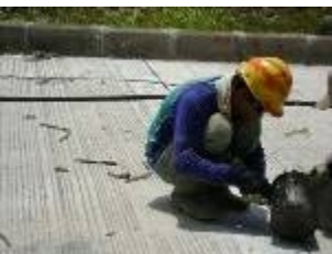
Underslab grouting, siap berfungsi 8 – 48 jam
