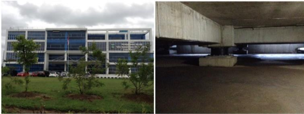
Fig. 18 – Seismic Bearing Installation
