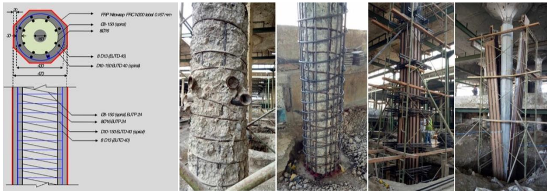
Fig. 11 – Concrete Retrofitting Design & Process
